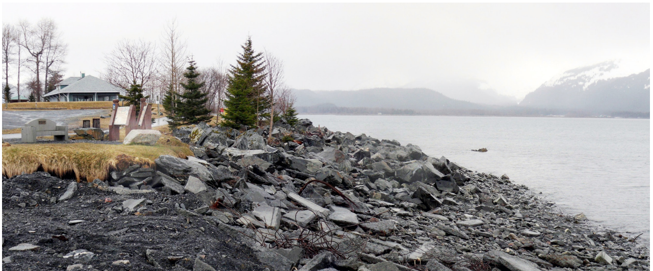
Fig. 2. Protection of the shore by concrete debris, Seward (Alaska). Photo by V. Afanasiev
