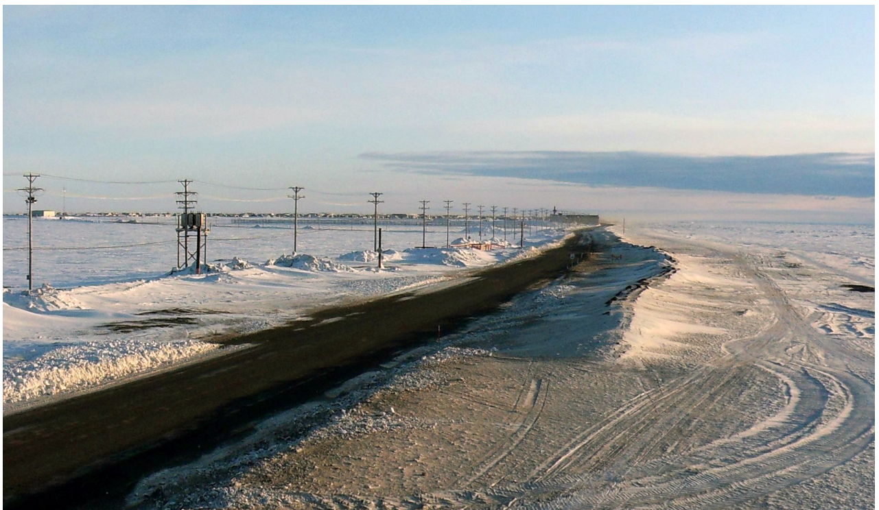
Fig. 3. Protective sand shaft, Barrow (Alaska). Photo by V. Afanasiev
